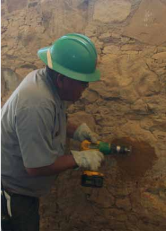
Figure 4. Operation of Electric Drill to Remove Graffiti from House Wall.
